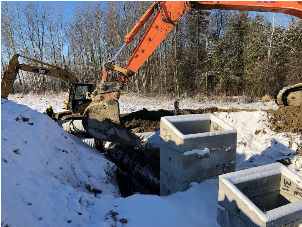
Installation of storm water infrastructure at rear storm water pond
