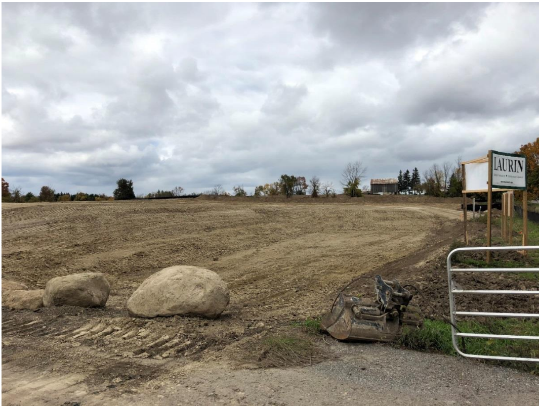
Construction entrance off Woodbine viewing North
