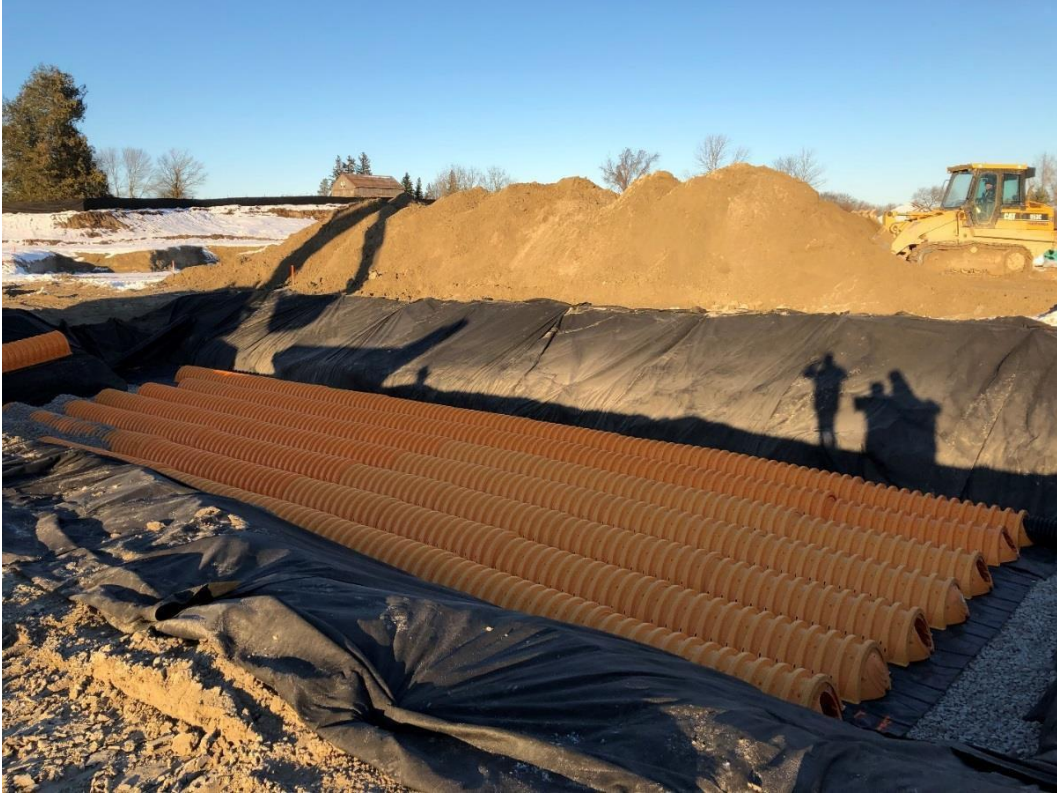
Site Servicing phase, installation of storm water infrastructure viewing North East
