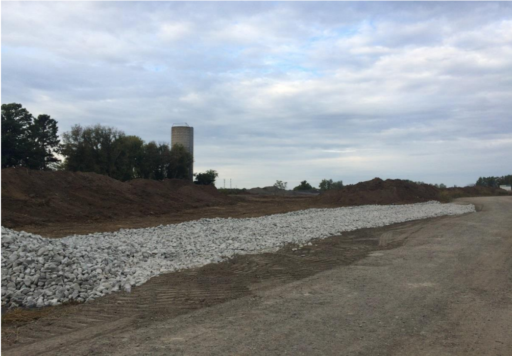
Construction entrance off Woodbine Avenue viewing West
