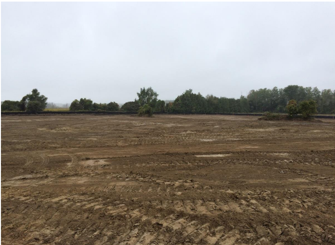
Grading and removal of fill viewing South
