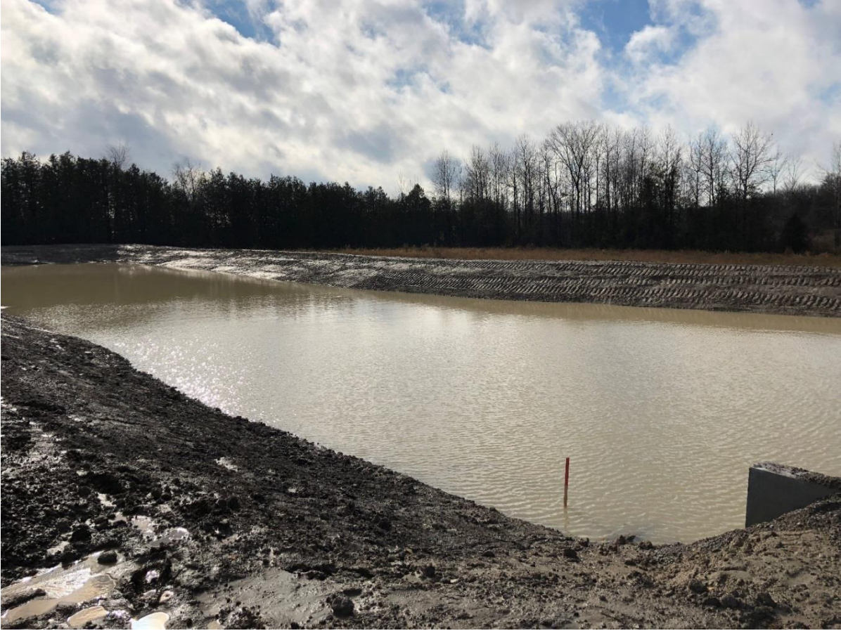
Storm water pond at rear of site viewing South West
