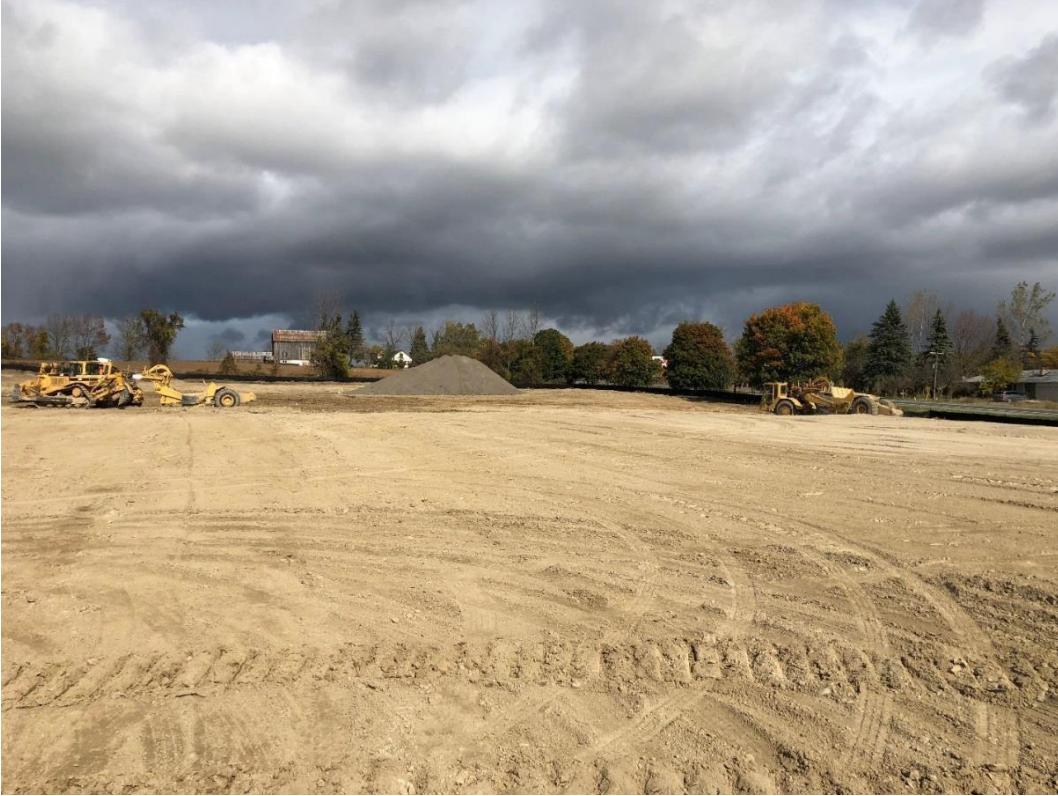
Grading and compaction of the future building site viewing North
