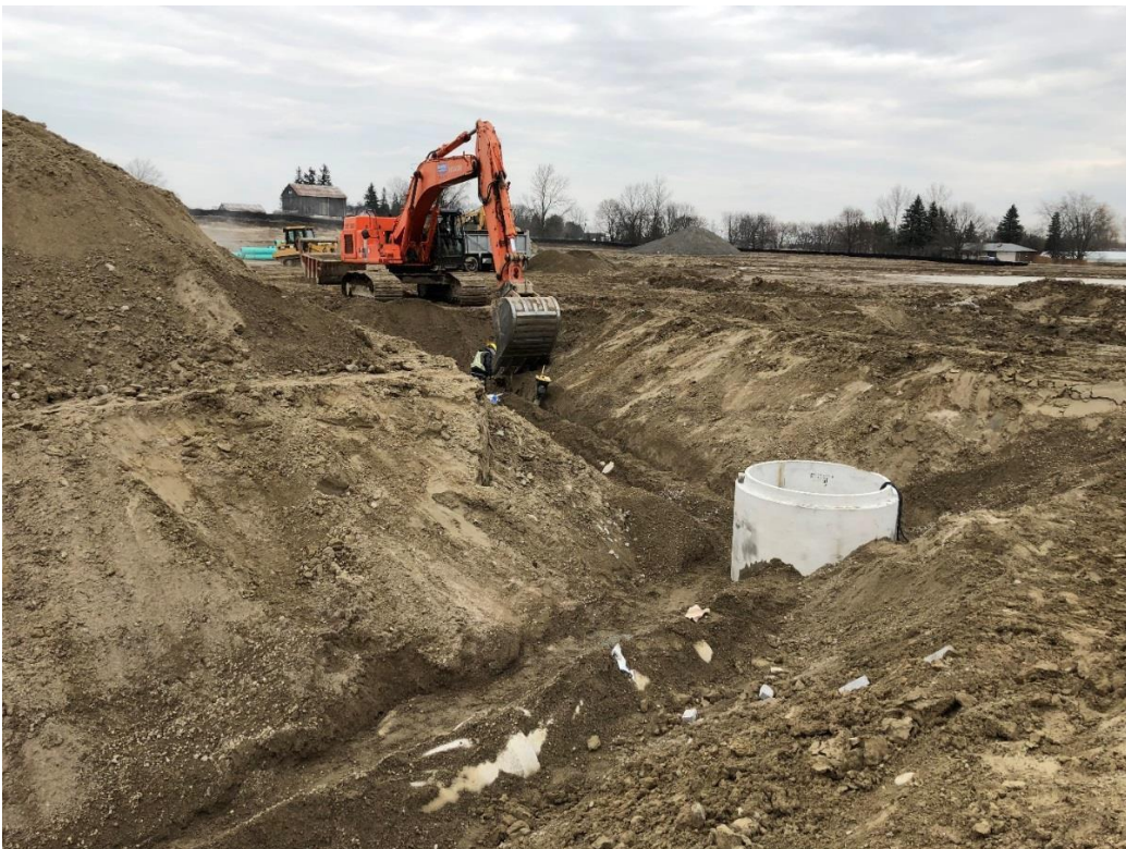
Site Servicing phase, installation of storm water infrastructure viewing North
