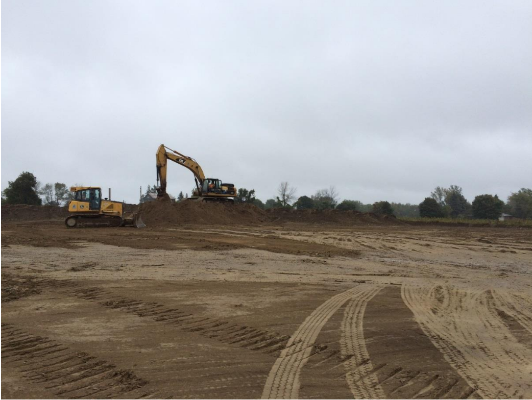
Removal of fill viewing North
