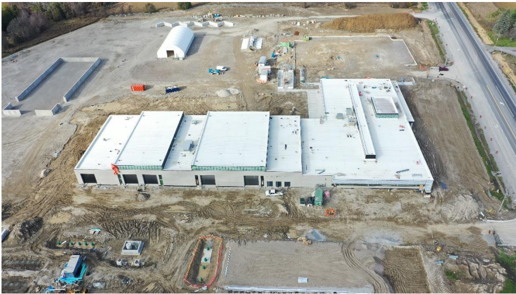
Operations Centre south elevation viewing to the north
