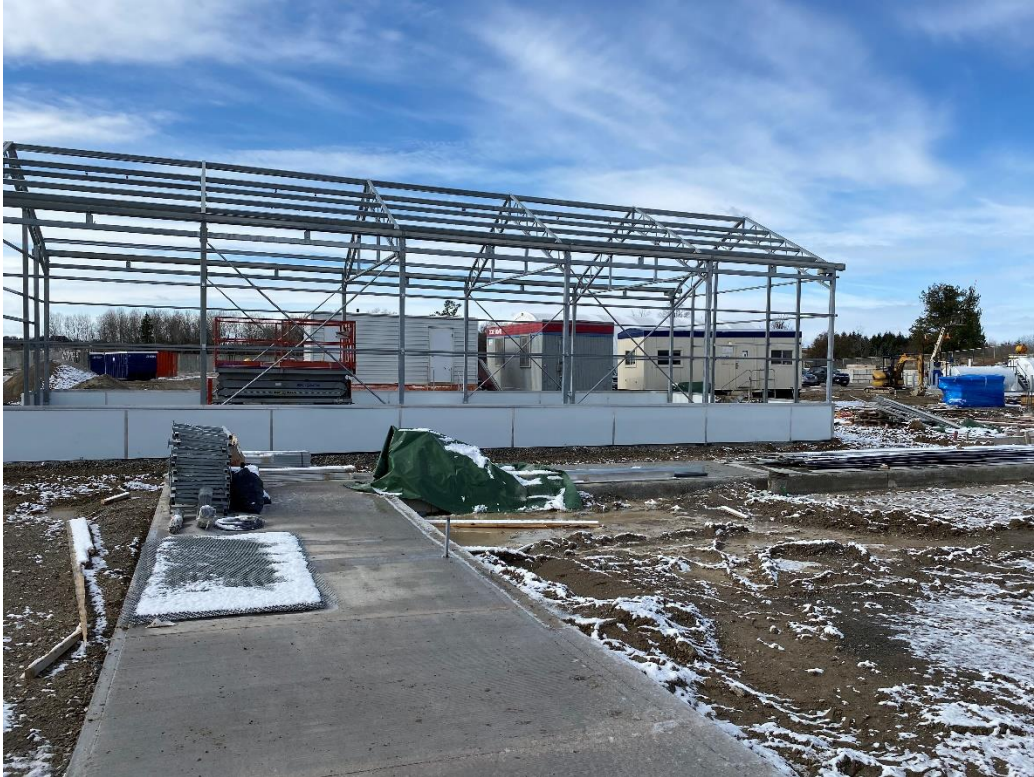
Structural steel and foam board shaping Greenhouse
