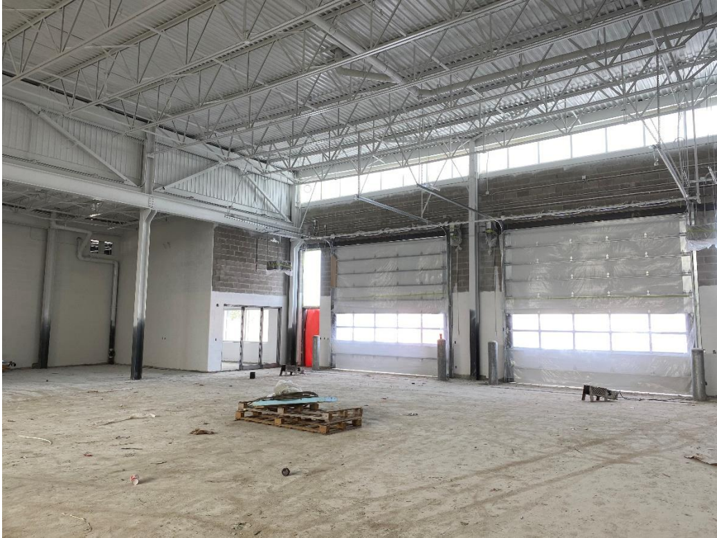
Painting of ceilings in Roads bays
