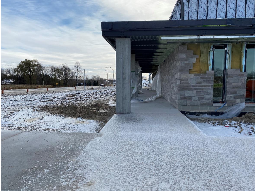
Concrete sidewalk from employee parking lot to front entrance
