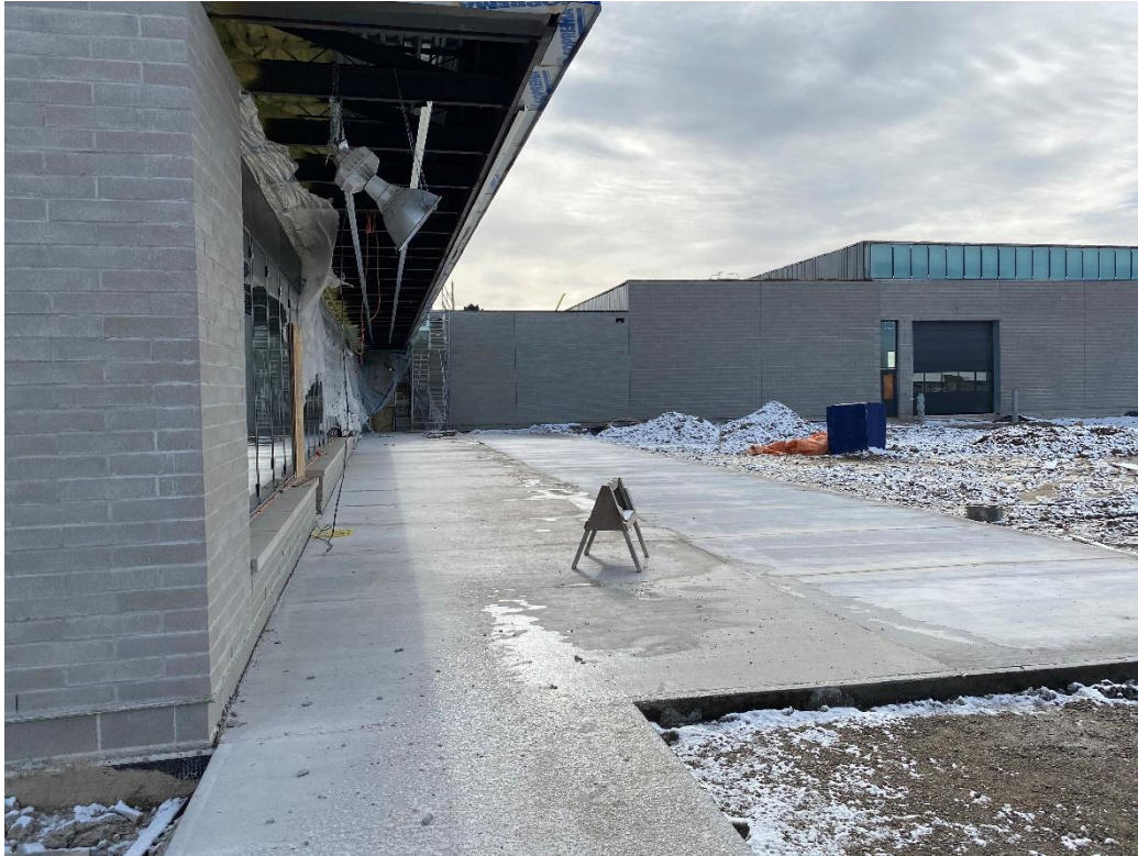
Concrete sidewalk from employee parking to field (staff) operator entrance
