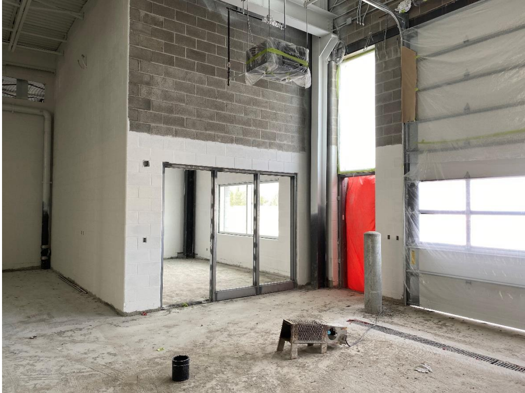
Framing and painting of Roads bay office
