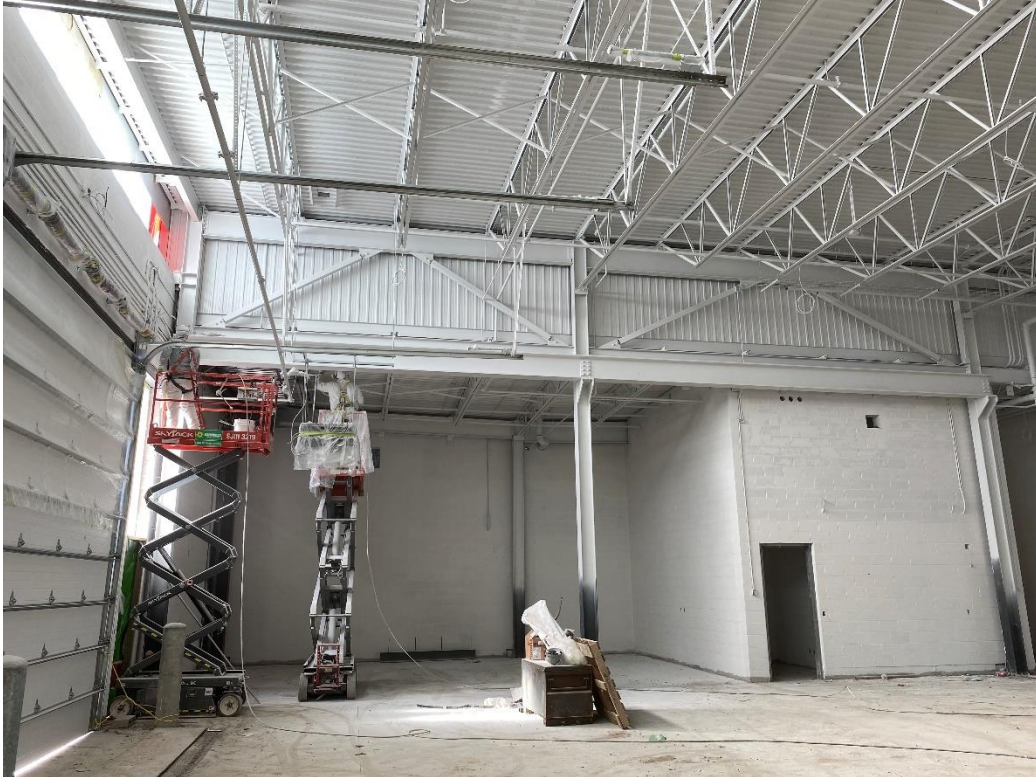
Painting of ceilings over the Roads bays
