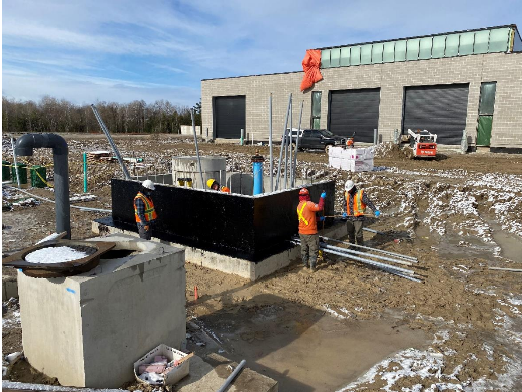
Fire water cisterns and pump house foundation
