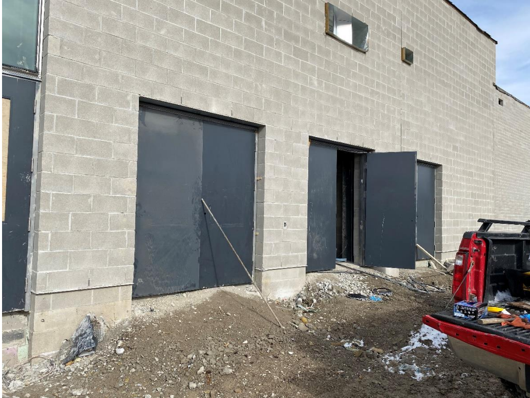
Frames and doors for Electrical and Sprinkler rooms south elevation
