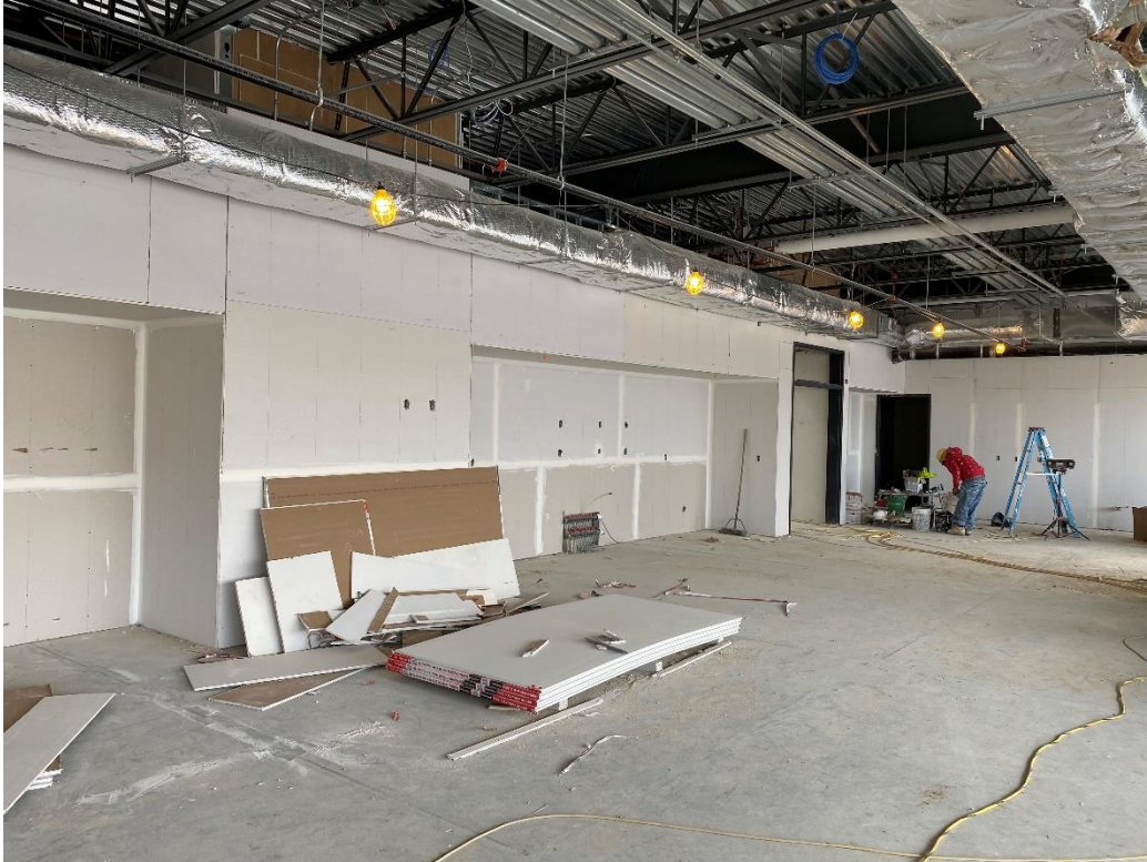
Drywall in the administration area Lunch room
