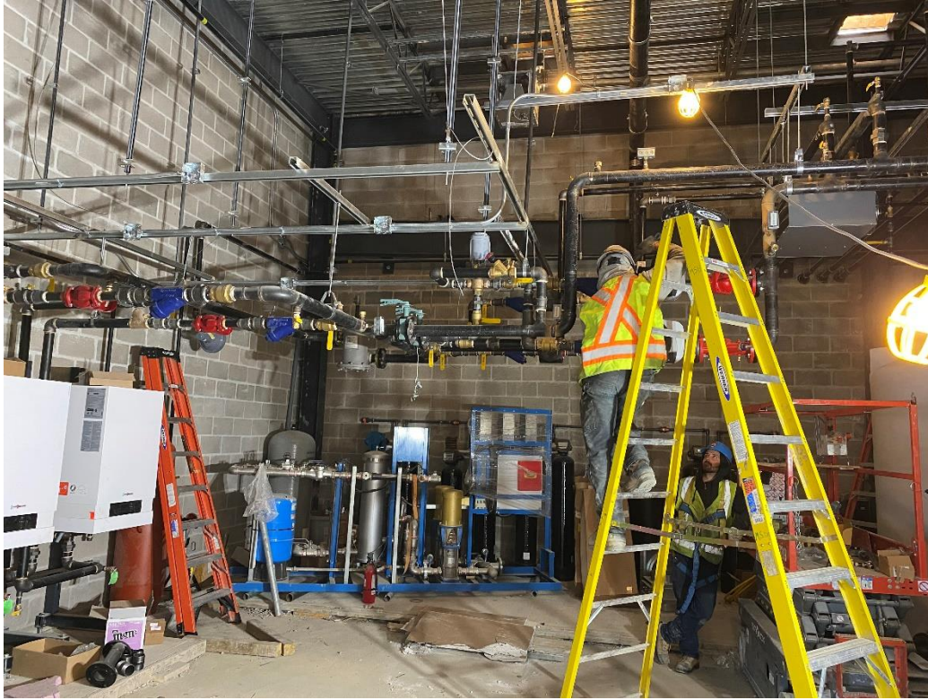
Installation, welding and piping of mechanical room
