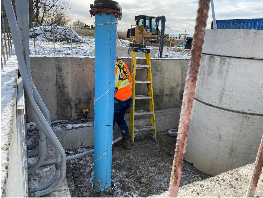
Fire water cistern pump house foundation and electrical conduit
