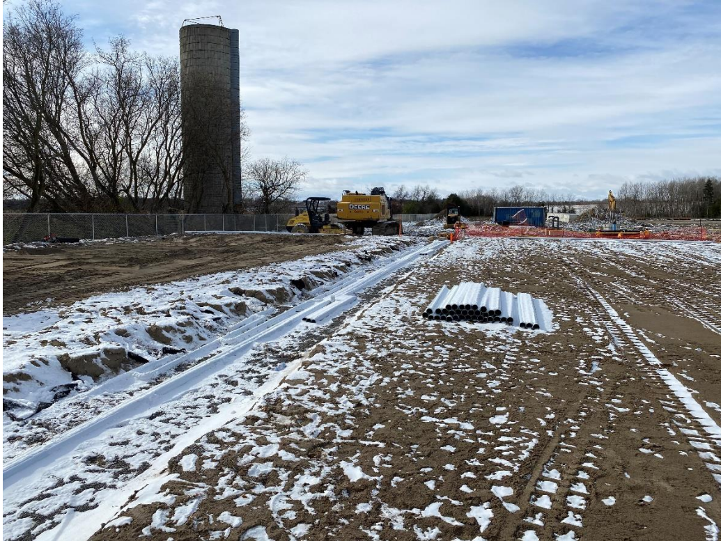
Installation of septic field piping south elevation
