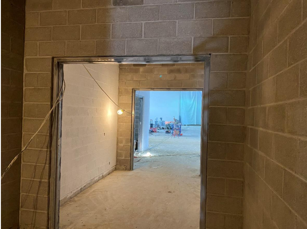
Interior masonry wall corridor leading to service bays
