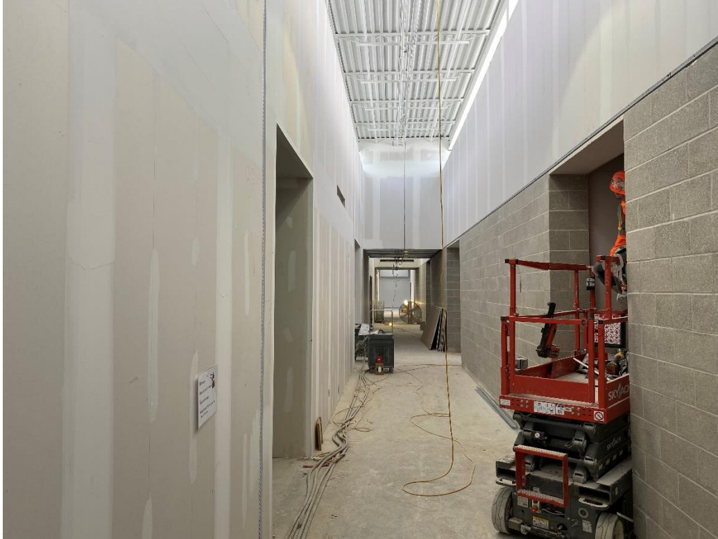
Staff north entrance corridor separating lunch room and meeting rooms
