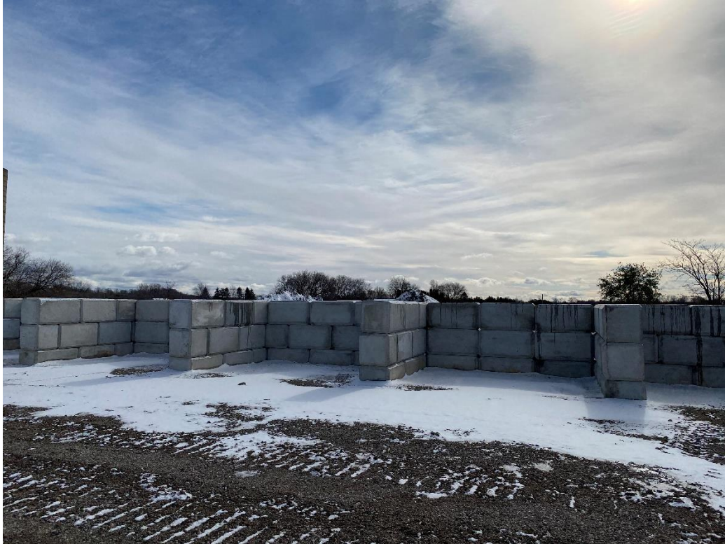
Retaining wall south part of site for mixed material supplies
