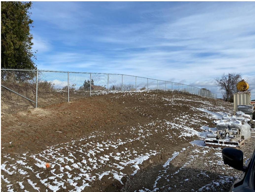
Installation of perimeter fencing along north property boundary
