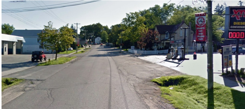
VIEW FROM MAIN STREET LOOKING EAST
