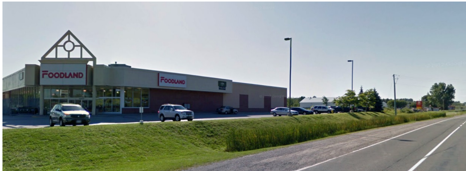
NEWER COMMERCIAL DEVELOPMENTS ARE FURTHER TO THE WEST, ALONG HIGHWAY No.48
