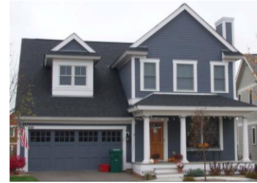
Figure 2.4.10.1a – Recessed Double-car Garage Door
