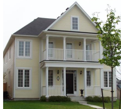
Figure 1.5.4 – Example of Architecture that reflects High Quality of Design
