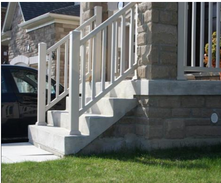
Figure 2.4d – Appearance of poured-in-place steps
