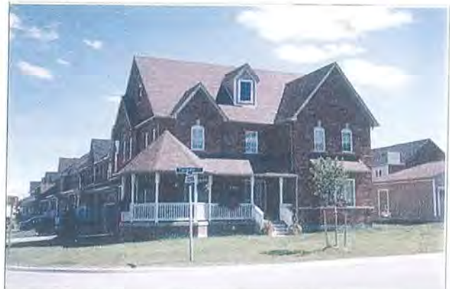
Corner house entrance
